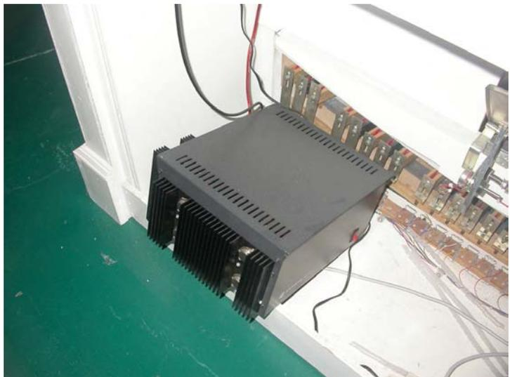
The new power supply. 70 Amps regulated at 12V.
